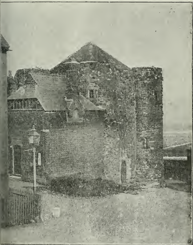
YPRES TOWER before removal of Soup Kitchen.
